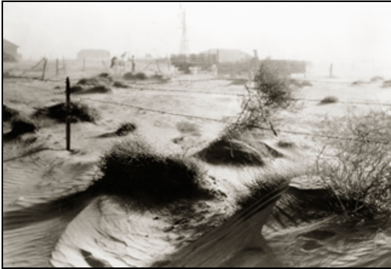
Dallas County, Texas, April 1938 (Farmstead damaged by sand drifting)
